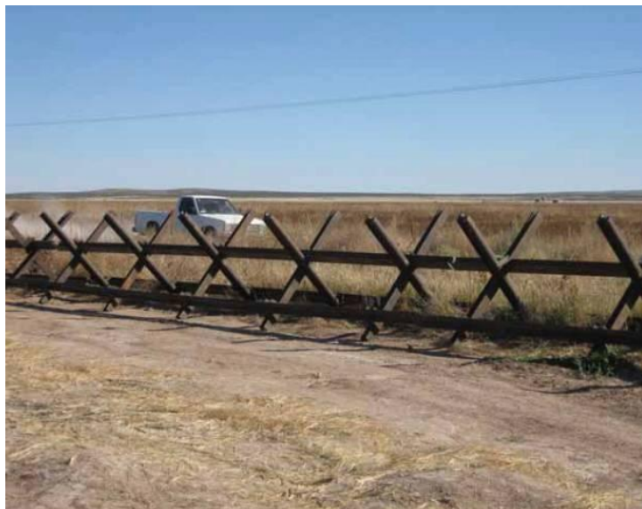
Figure 21: Normandy style vehicle barrier Photo by AGFD / Duane Aubuchon
