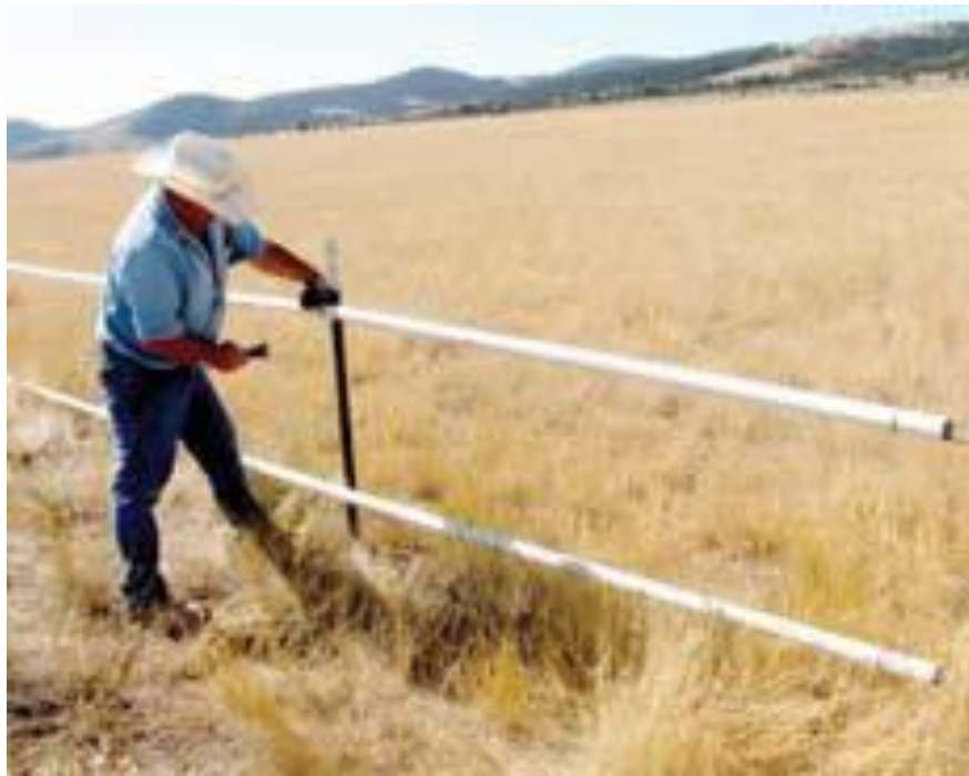
Figure 11: Installation of crossing structure: Note the plastic pipe slipped around the top and bottom wires
